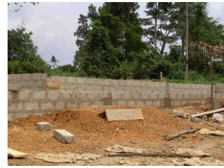
Foundation work in progress
